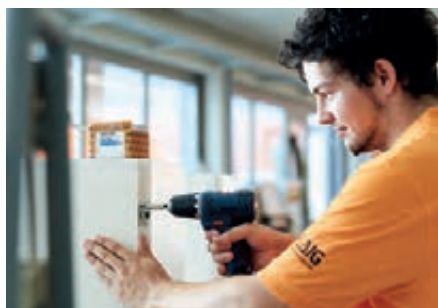
Installation of fittings on ends of boards
