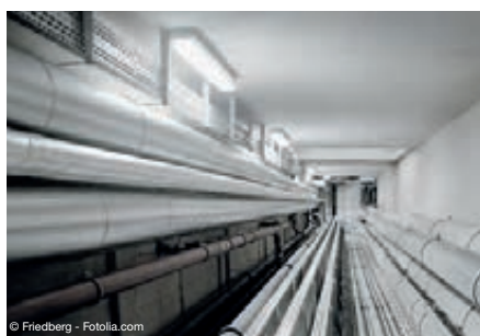
Fixing of cable ducts
