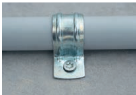
Fixing of cable clamp
