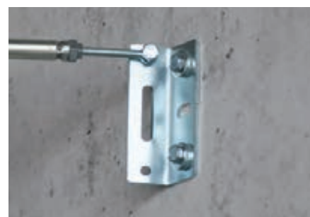
Fixing of brackets and console bearers
