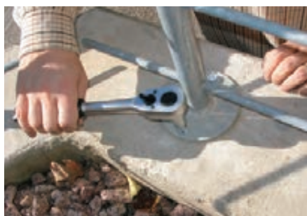
Fixing of railing
